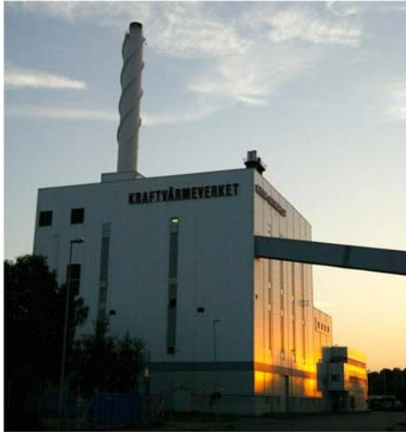
Figure 8: The ENA powerplant in Sweden (left) and the gypsum additive used in ENA
